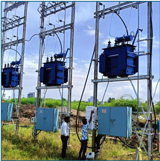
Installation of Transformer & Switchyard, West Bengal
